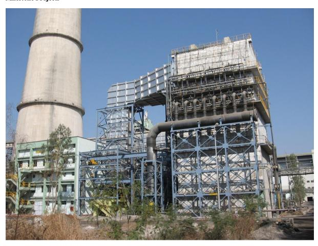
(India's first Sea water FGD system with 100% of flue gas, for 2 X 250 MW DahanuTermal Power Station at Dahanu, Maharashtra, India installed by Ducon)
